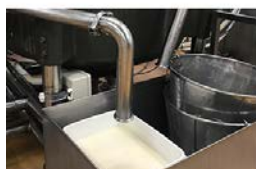
The mayonnaise discharged from piping when shifting production from one product to the next
